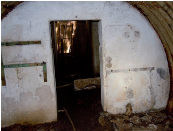
The main chamber inside the underground Harrietsham Zero station
